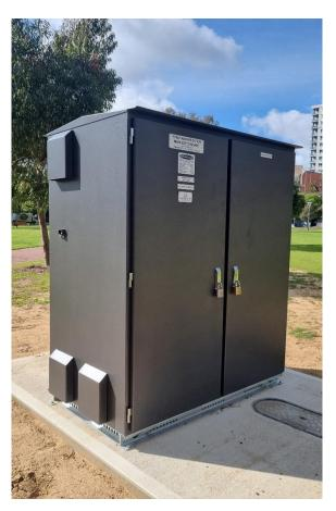
The Light Square Electrical Major Switch Board was upgraded to facilitate a 300amp supply to the area. This upgrade will support events such as Fringe and Illuminate in this space and potentially increase revenue.
