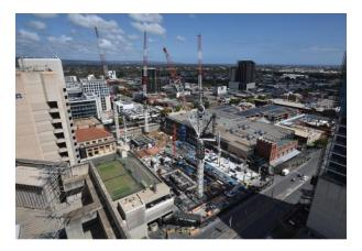
In the last quarter, major progress has continued on site including the completion of the basement excavation and retention works to the lower basement levels. This has involved the removal of 83,000 tonnes of soil material from site in total.
